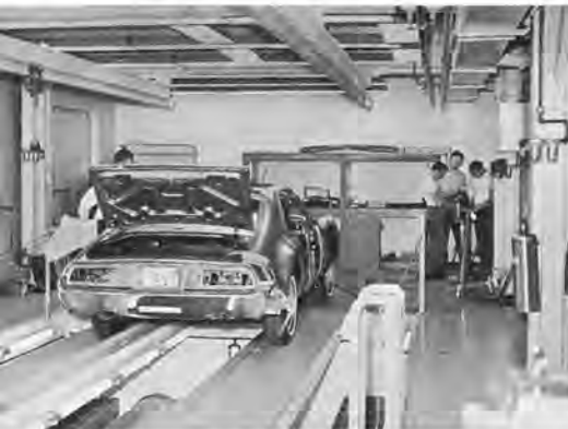
Fig. 11—LABORATORY TESTING OF ASSEMBLY OPERATIONS. The facilities of Oldsmobile's laboratory used to finalize assembly planning for the Toronado included conveyor sections, fixturing, and tooling (top). Of particular importance during the laboratory testing phase was developing the final methods for setting the Toronado body onto the frame (center). The laboratory also provided facilities for tryout of final assembly line operations including center and outboard pits (bottom).
